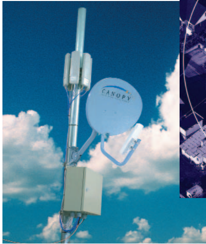
The Access Point (center) sends information to and from the Backhaul Unit (left) and the subscriber module (right) located on the customer's premises.
