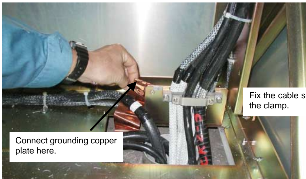
Fig. 1-26 Grounding chassis
