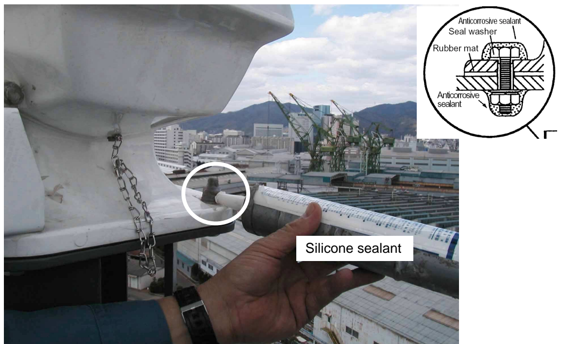
Fig. 1-4 Applying silicone sealant
