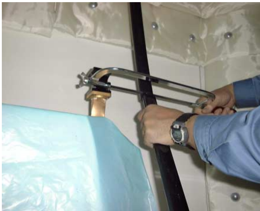
Fig. 1-18 Cutting waveguide
