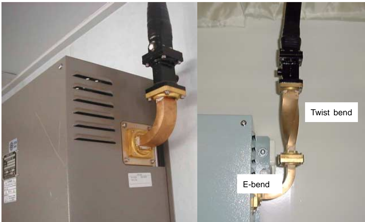
Fig. 1-24 Connecting waveguide to transceiver
