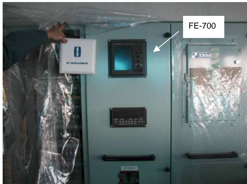
Fig.5-48 Installation of FE-700 echosounder
