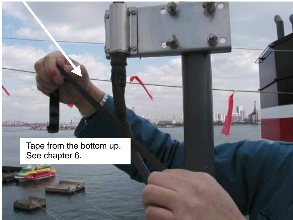
Fig. 3-12 Waterproofing of antenna connector
