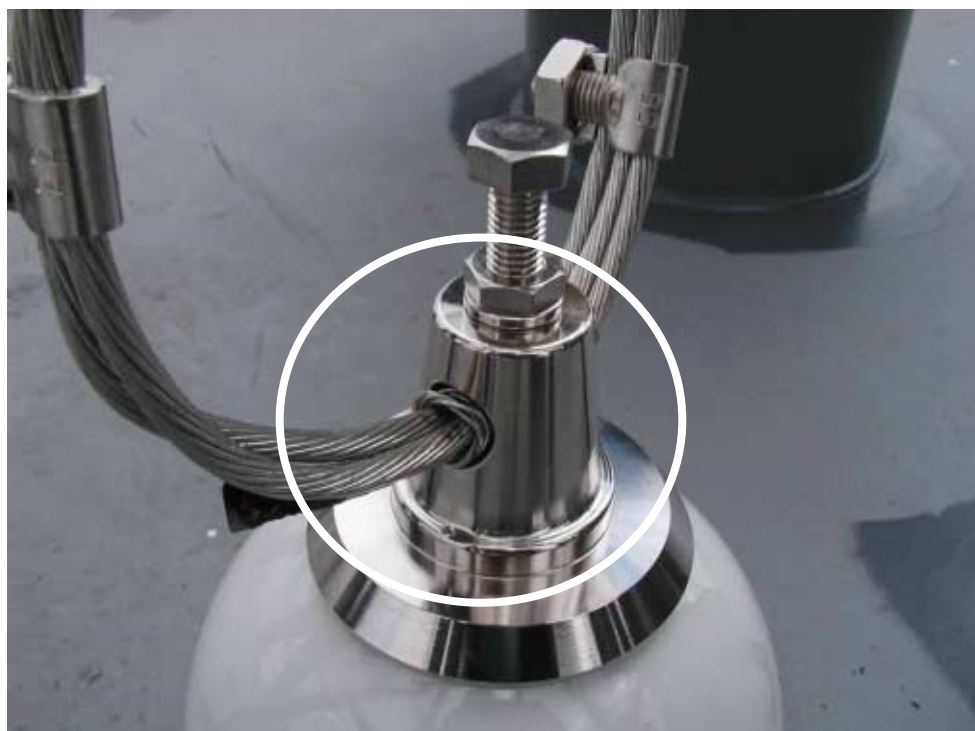
Fig. 3-6 Fixing antenna wire
