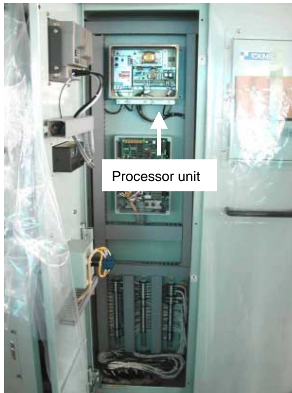
Fig.5-50 Installation of FE-700 processor unit
